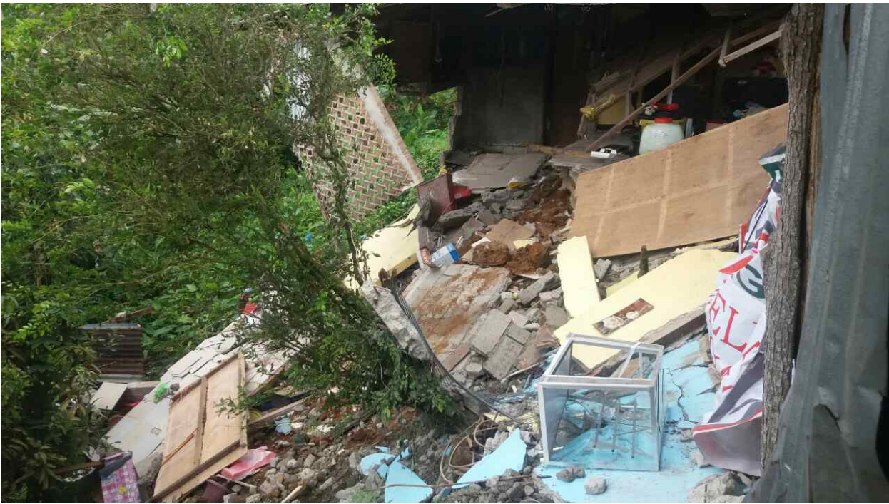
Photo 4. Damaged house in Brgy. Danao, Ormoc City. (Photo by: LCDE)
