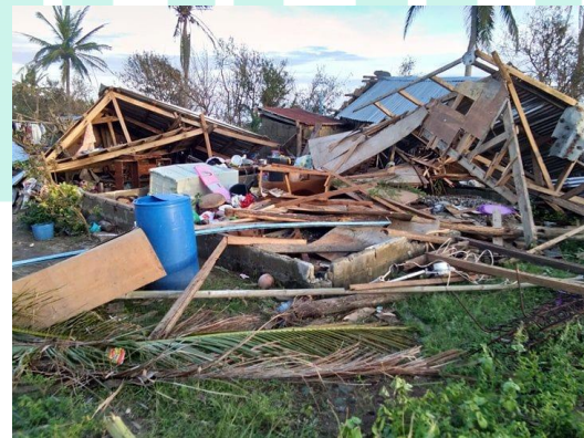
Destroyed houses in Talisay, San Narciso, Quezon
