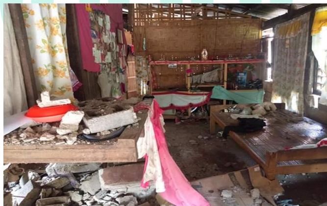
M6.3 earthquake aftermath in Magsaysay, Davao del Sur
